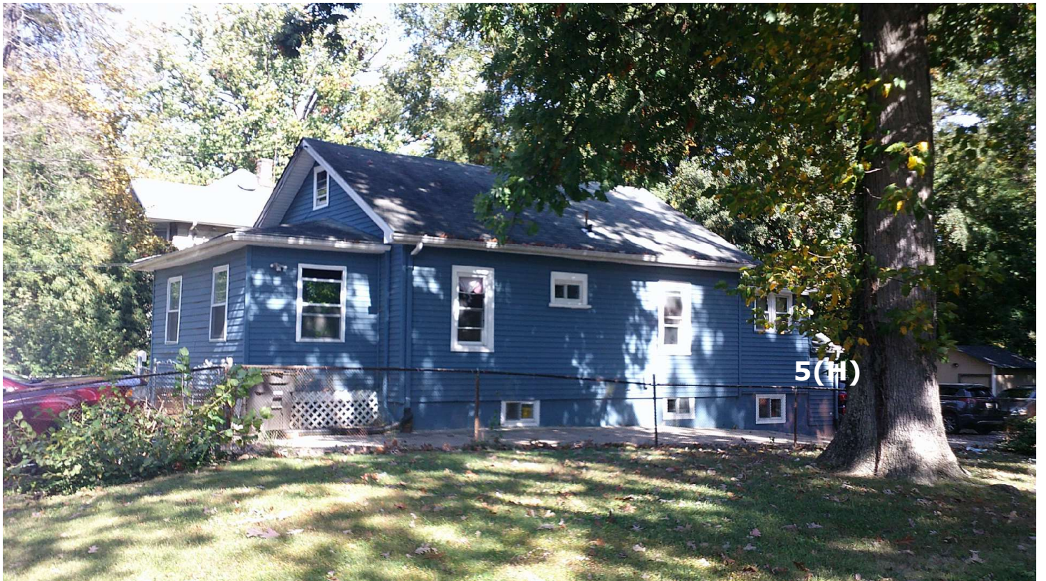
FRONT RIGHT VIEW FROM NEXT LOT
