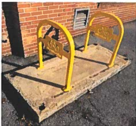
Completed bike rack installation:
