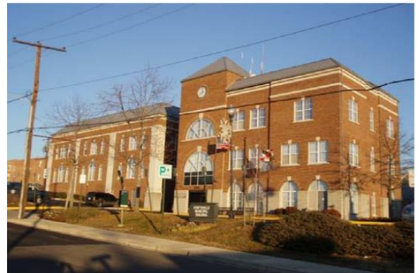
Photograph 1. Hyattsville Municipal Building
