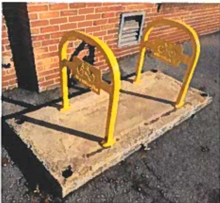
Completed bike rack installation:
