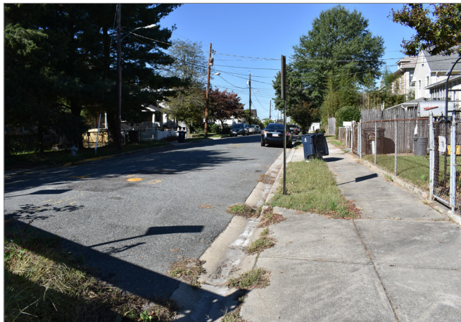
Figure 41. Existing right-of-way conditions
