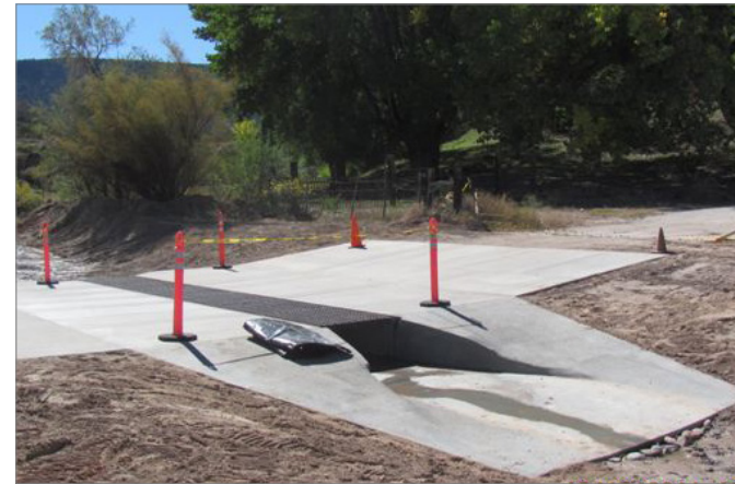
Figure 28: Example of a water crossing
