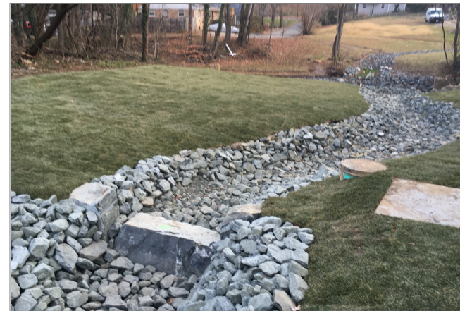
Figure 18. Outfall stabilization project in Suitland, MD
