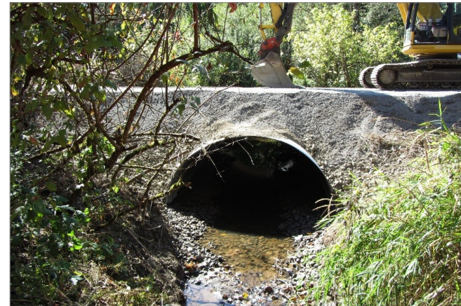
Figure 26: Culvert replacement project under a park trail
