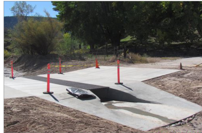
Figure 28: Example of a water crossing
