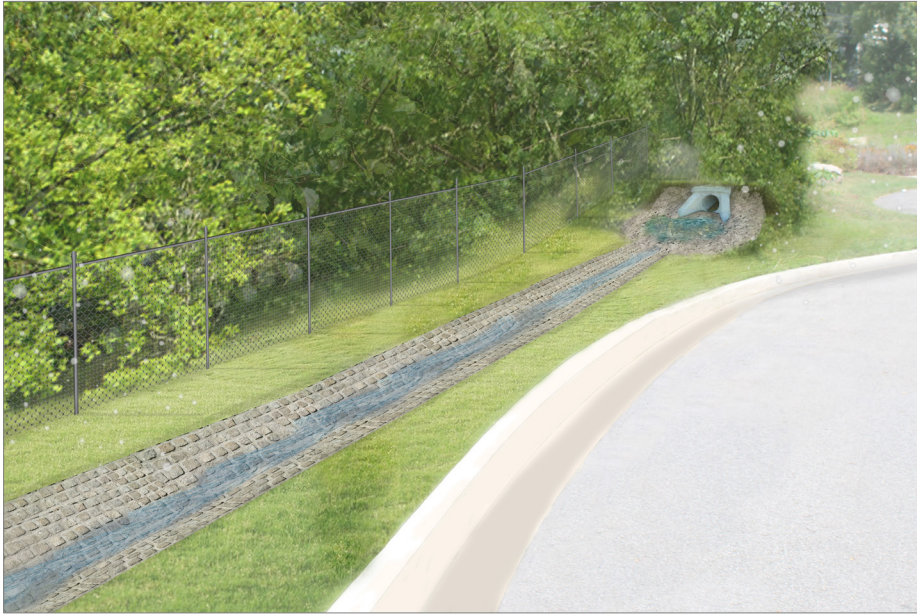
Figure 19. Rendered overlay of 41st Street outfall restoration project. A plunge pool is installed directly below the outfall.
