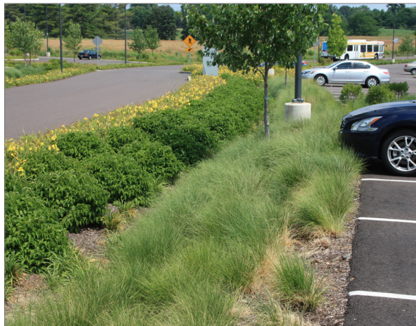
Figure 33. Bioswale along edge of hospital parking lot in East Norriton, Pennsylvania
