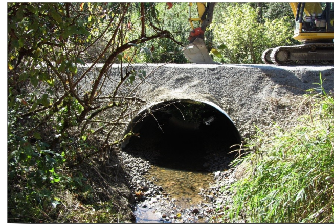
Figure 26: Culvert replacement project under a park trail
