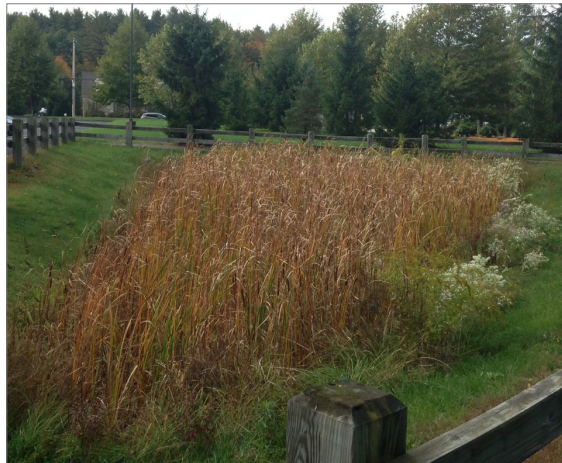
Figure 31. Example of a submerged gravel wetland
