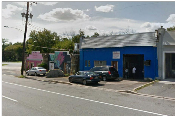
Figures 29. Existing curb-and-gutter along Rhode Island Ave southbound
