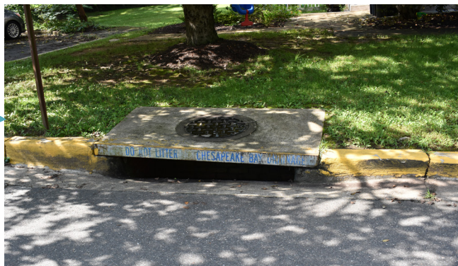
Figure 15. Existing storm drain inlet along 41st Place
