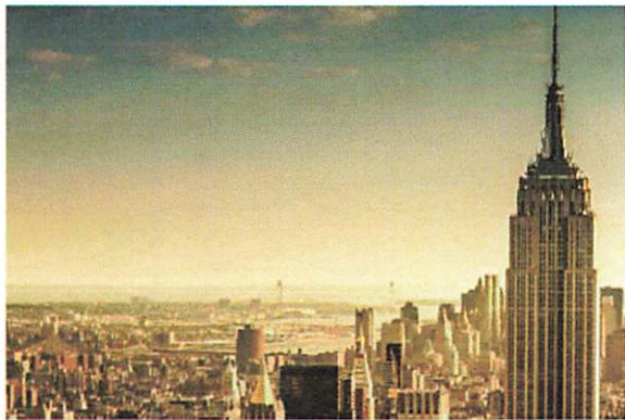
Our Systems Protect Many of the Most Iconic Buildings in America, Including the Empire State Building.
