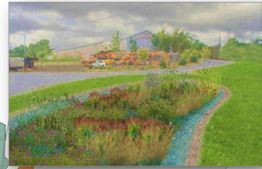
9 Submerged Gravel Wetland
