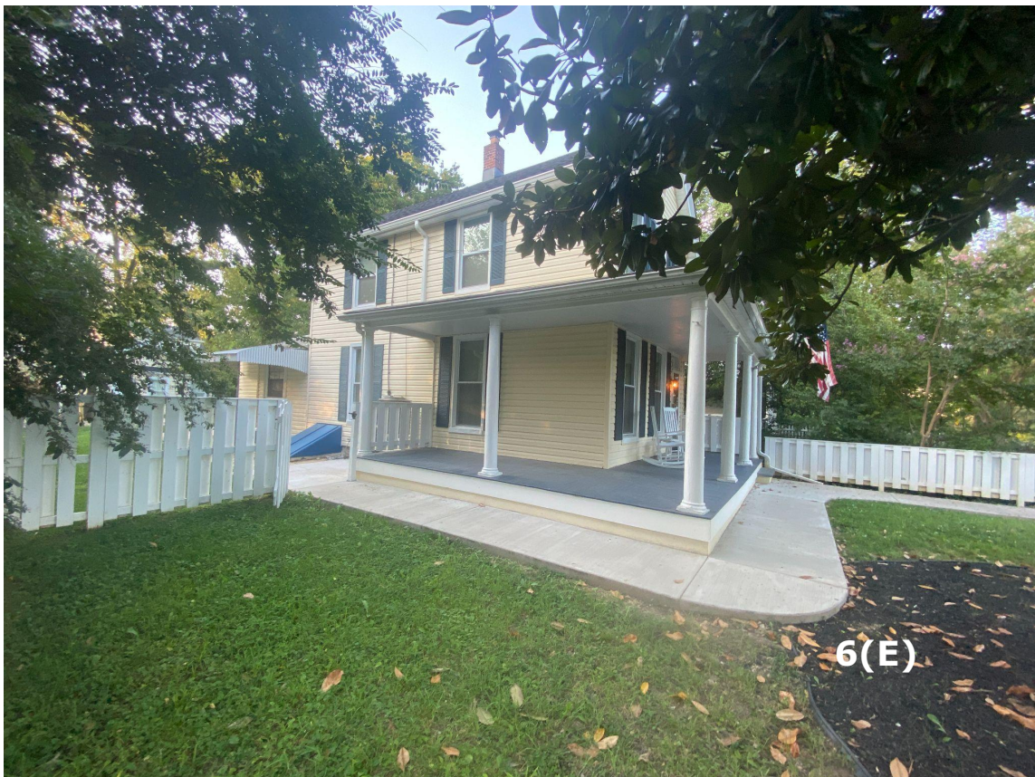
SIDE YARD VIEW #2
