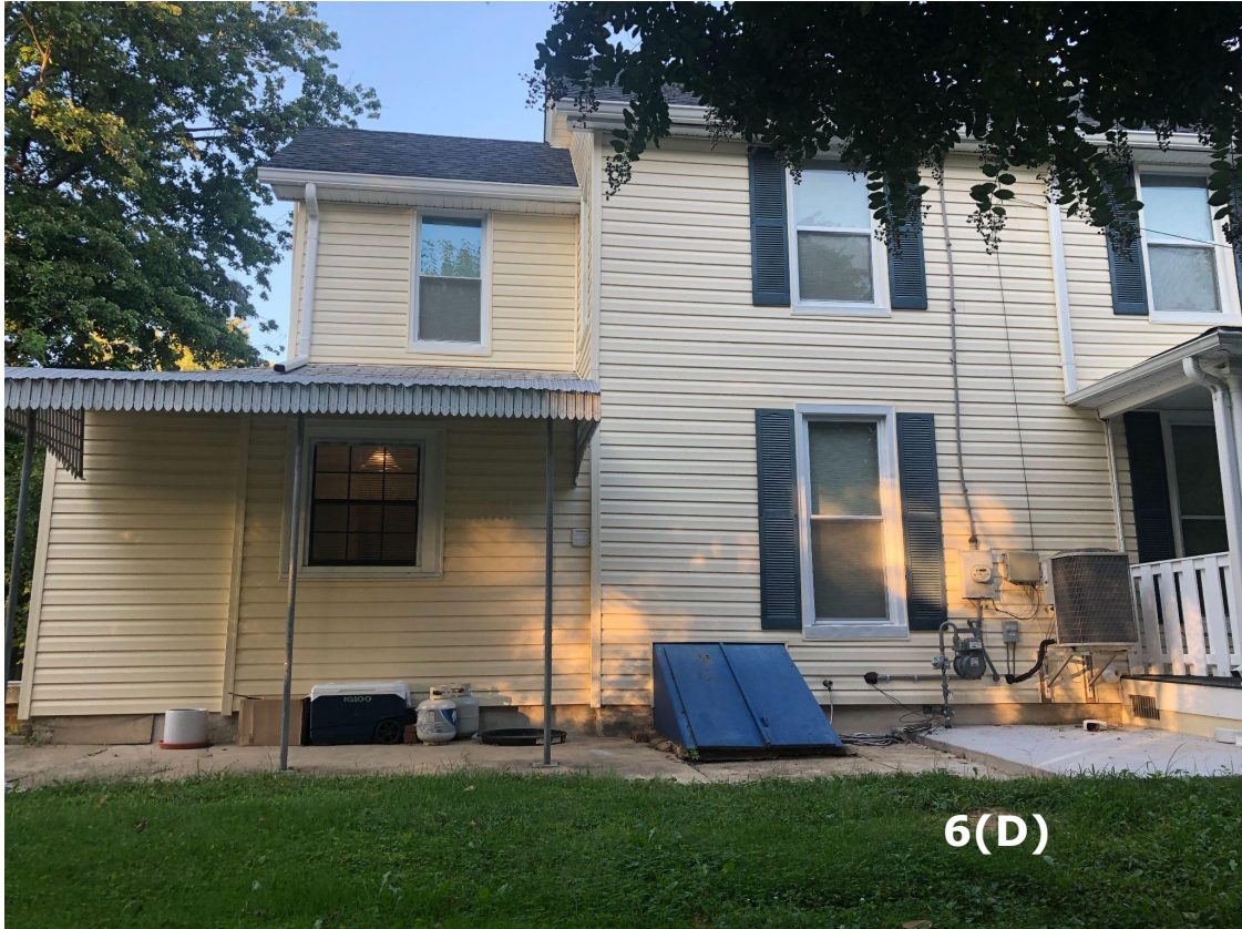
SIDE YARD VIEW
