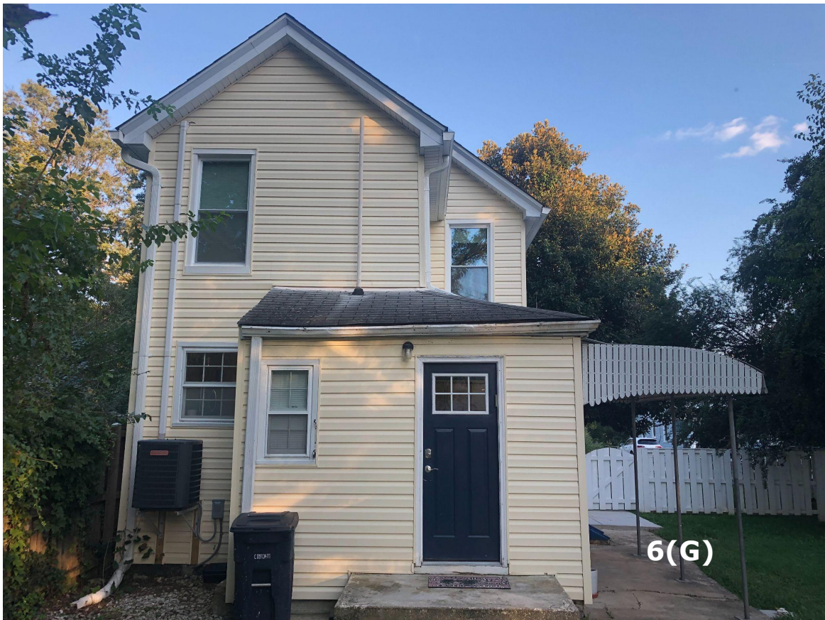
REAR OF THE HOUSE
